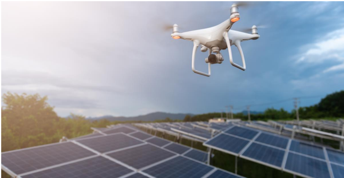
Figure 25: Solar PV plant inspection using drones
