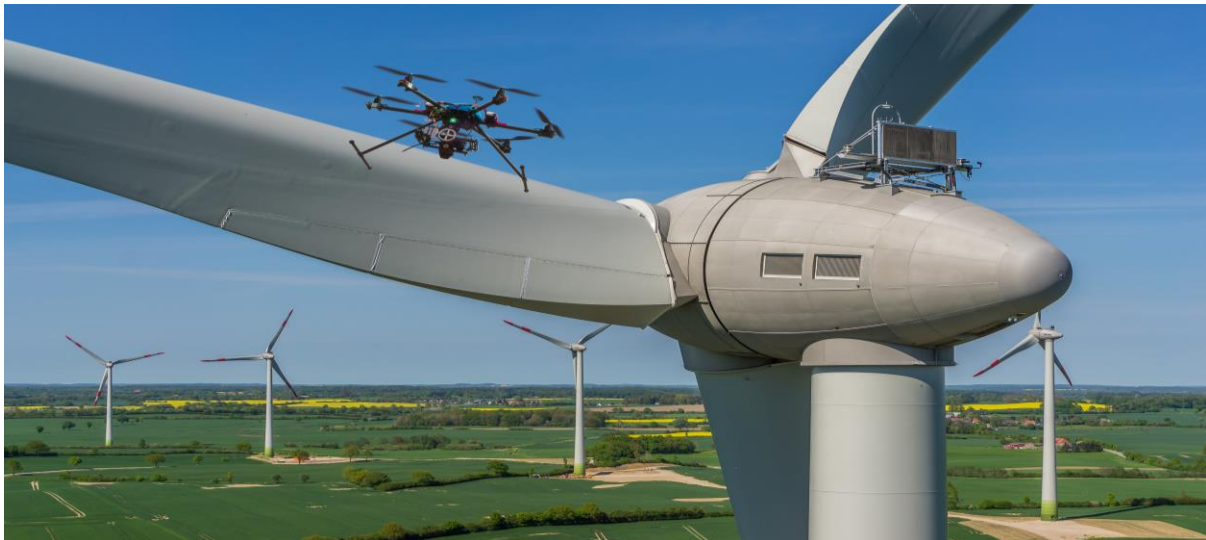
Figure 27: Wind turbine inspection using drones
