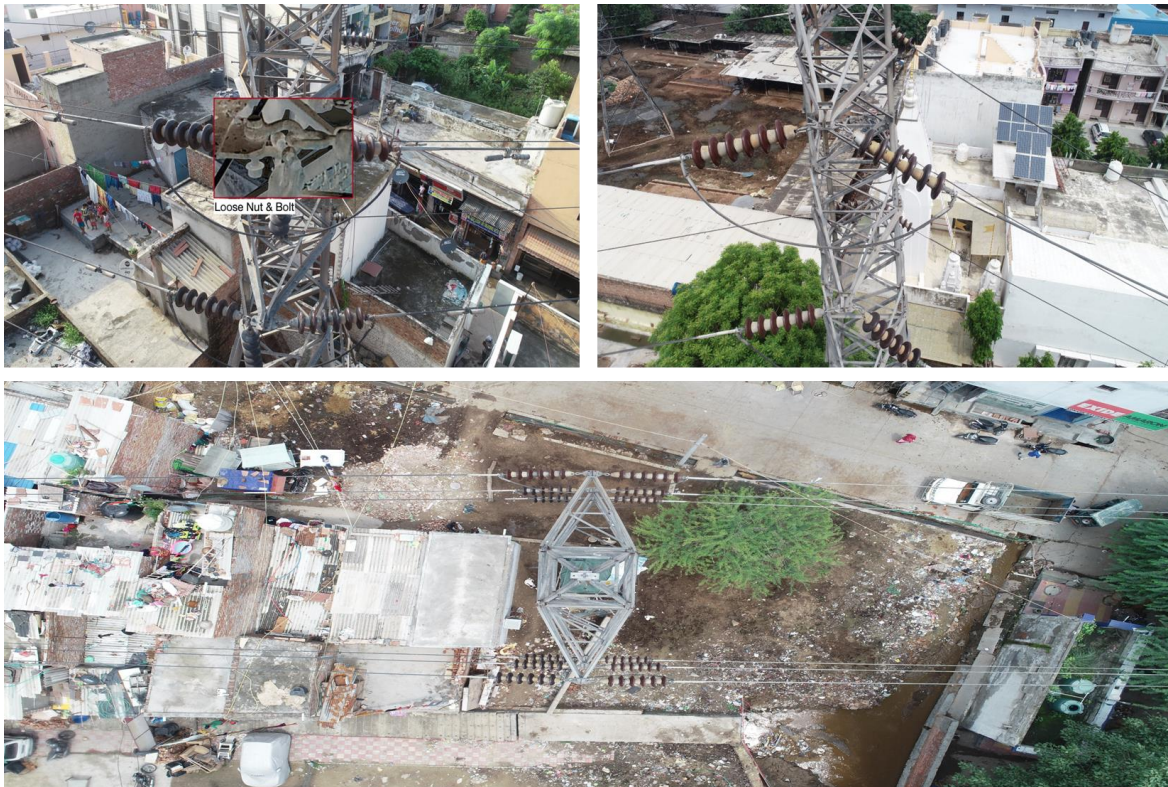
Figure 6: Sample defects
