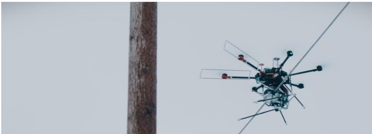
Figure 14: Installation IoT sensor on power line by autonomous drone
